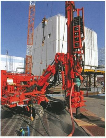
Drilling of the first of 1550 holes has started at Fukushima Daiichi (Image: Tepco)
